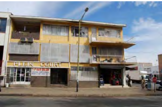
4: Poor Condition around Taxi Ranks
