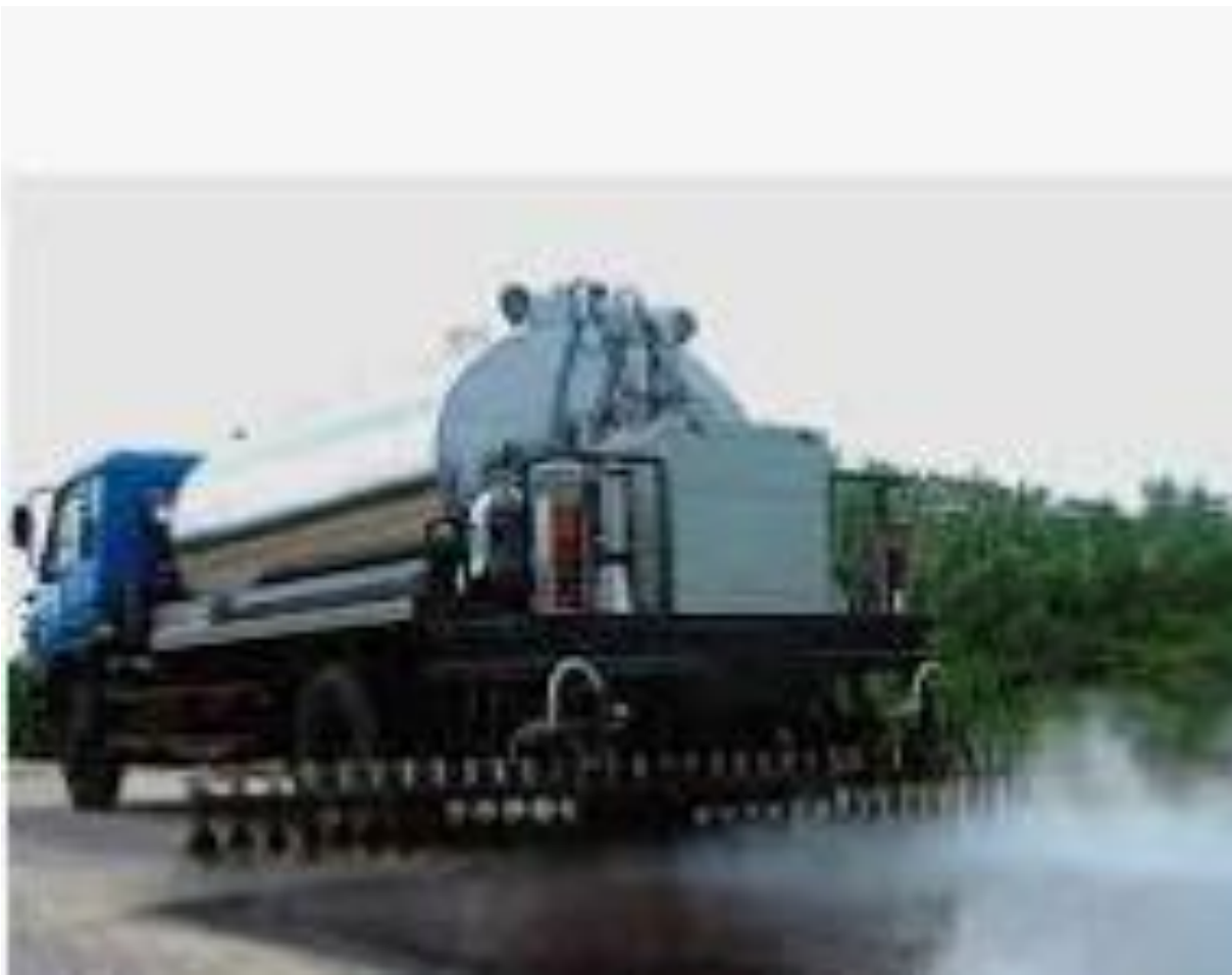
Application, using a spray tanker (Cationic Emulsion)
